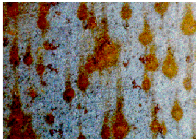
FIGURE 4 - Corrosion Damage to Unsealed HVOF WC/Co Coating
